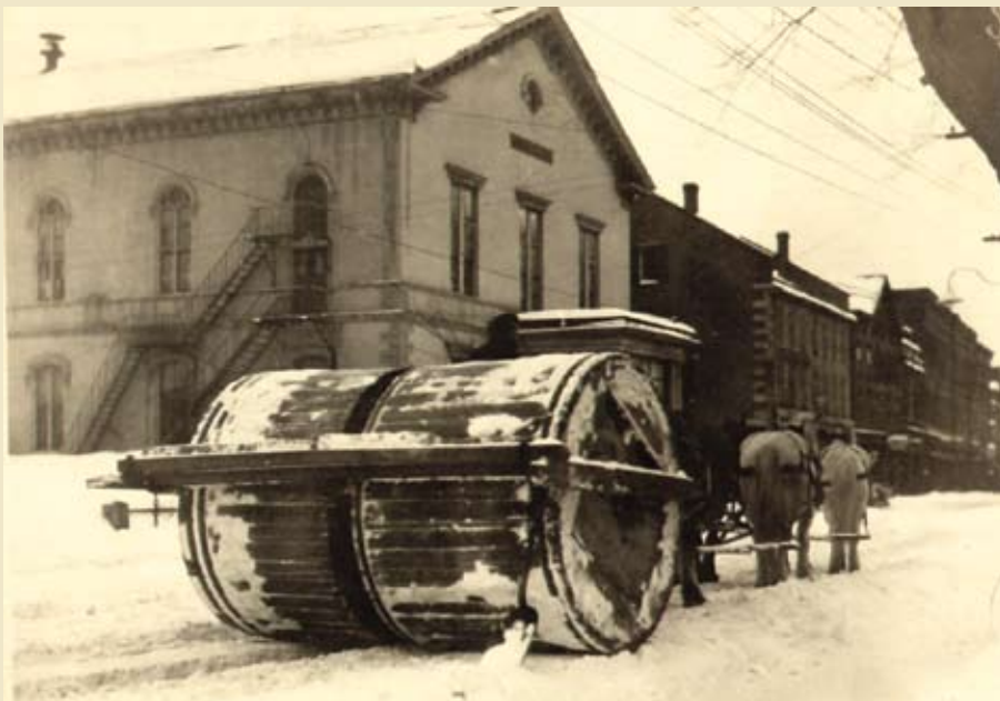
Historical photo of a snow roller in use on Main Street in Brattleboro, Vermont, circa 1920's, early 1930's. Photo Courtesy of Brattleboro Historical Society in Vermont.
